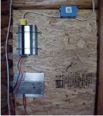
Power Panel with Inverter and Charge Controller
