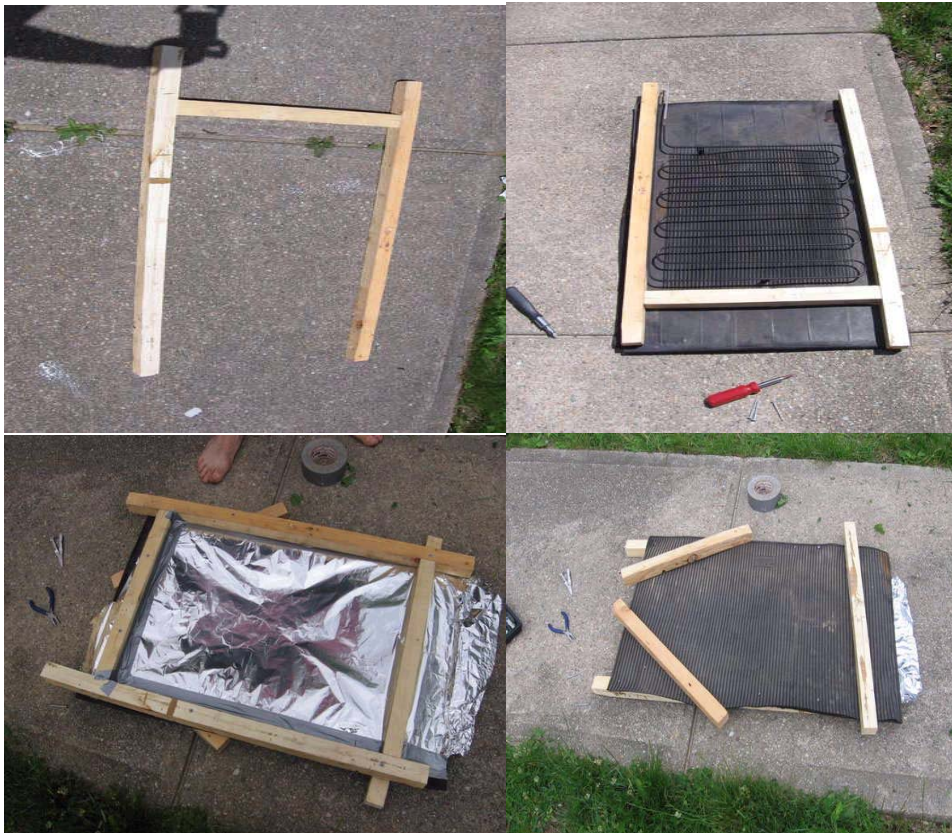
Attaching Collector To Frame
