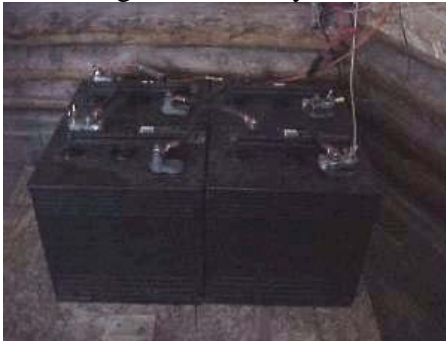
Battery Bank -- 4 Golf Cart Batteries
